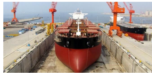
Gambar 1. Dock Kolam ( Graving Dock )
