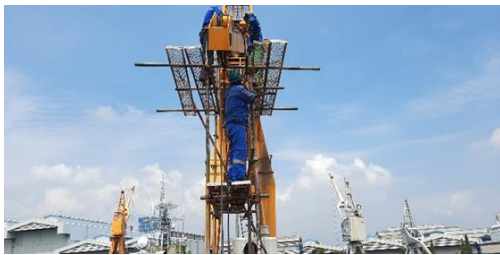
Gambar 18. Slewing Lengan Floating Dock Crane
